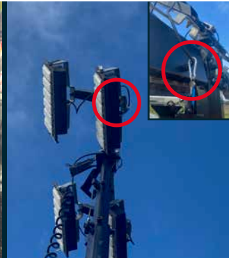
2. Teether key(s) to top of mast (insert) and raise.
